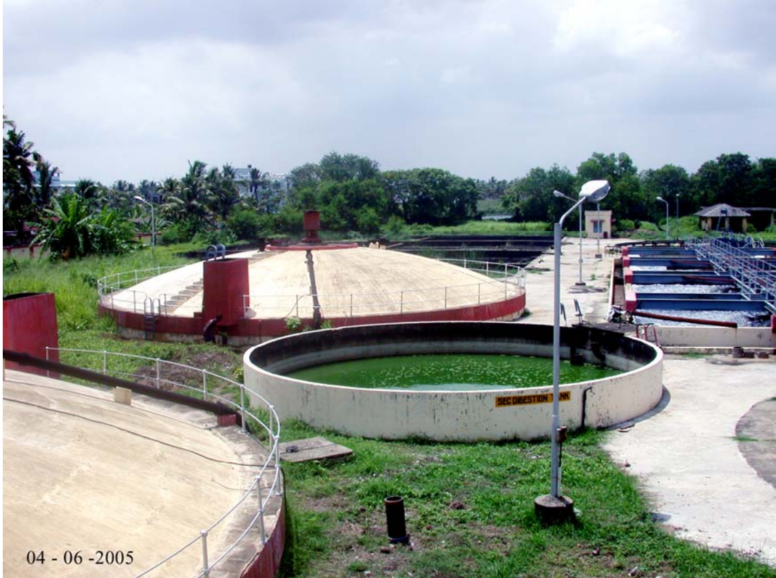
Figure 1.5: Another View of the Treatment Plant (Existing)
