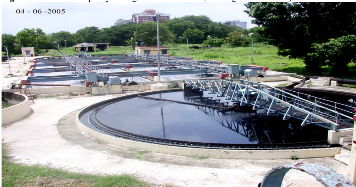
Figure 1.4: 4.50mld Capacity Sewage Treatment Plant (Existing at Elamkulam)
